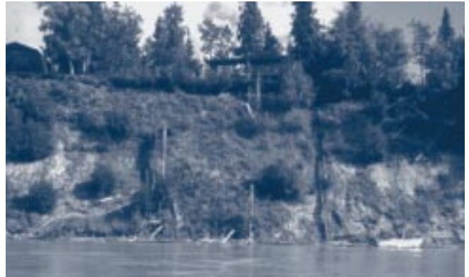
This bank is too steep and the material is too loose to be stabilized by vegetation or anything else. Erosion here is inevitable.
